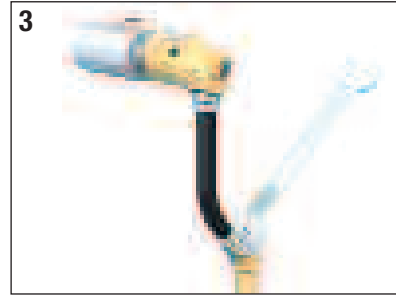
3 Connect flexible hose to supply line.
